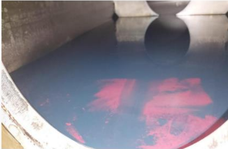
195 DMU – Inside the tank (black dust)
