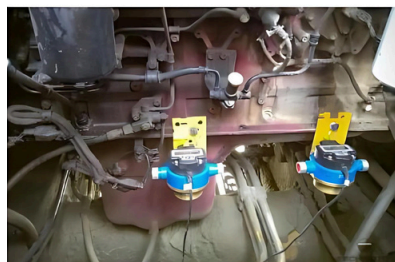
Installing fuel flow meters on front engine of Komatsu
